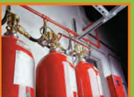
For applications in which the materials involved are subject to smoldering fire conditions, Fike's **CO<sub>2</sub>** system provides a heavy blanket of agent which penetrates all parts of the vessel, quickly extinguishing these deep-seated fires. And unlike water, there is no clean-up necessary with a Fike **CO<sub>2</sub>** system discharge, for minimal interruption to your business!
